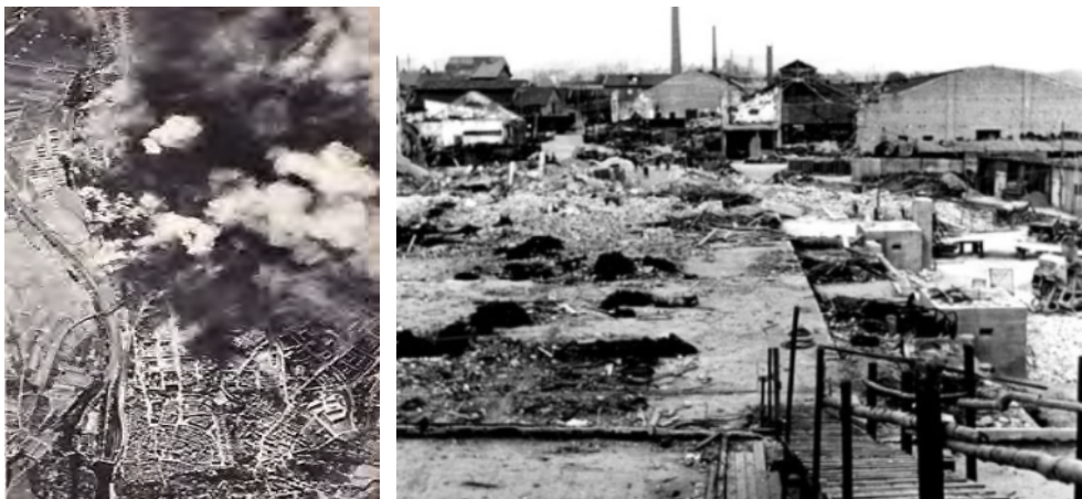
Bombardment of Schweinfurt Destroyed ball bearing factory, Schweinfurt, October 1943
